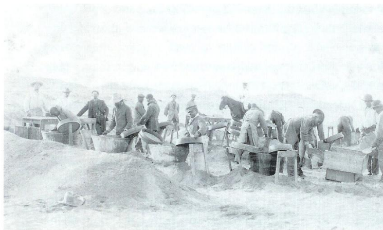
Figure 8: Photograph depicting early mining methods (c.1911/13) Note that digging and washing done entirely by hand. (Sam Cohen Library, Swakopmund)
