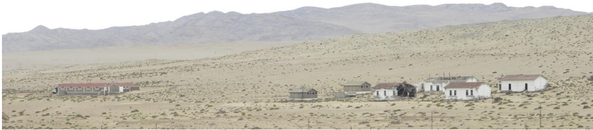
Figure 32: Segregated Living Quarters Omtanda (Left) and 'Native' Compound (Right) (N Alexander, 2010)
