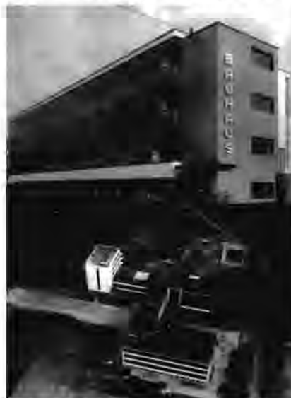
Figure 2: Bauhaus building in Dessau Germany, by Walter Gropius (1926)
