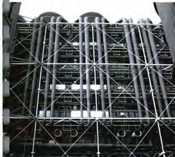
Figure 105: Photo of exterior services on facade of Pompidou Centre
