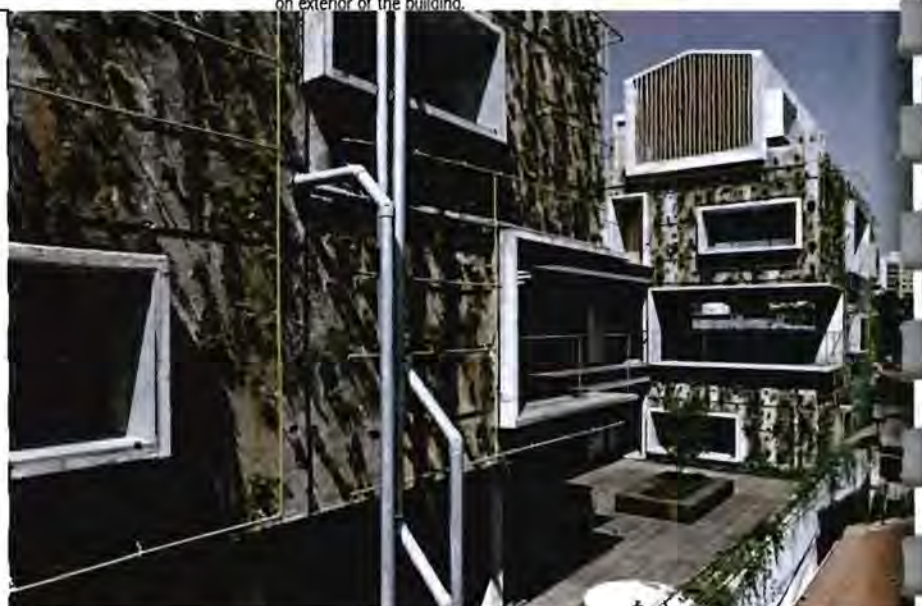
Figure 103: Photo of Harmonia 57 with vegetation & water reticulation on exterior of the building.
