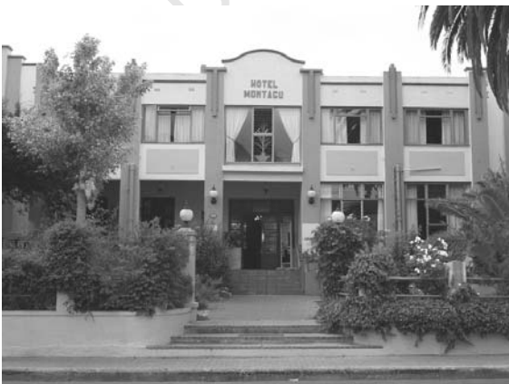
Figure 10: The Art Deco, 1930s Montagu Hotel (now the 'Montagu Country Hotel'), on Bath Street, originally a Victorian building.
