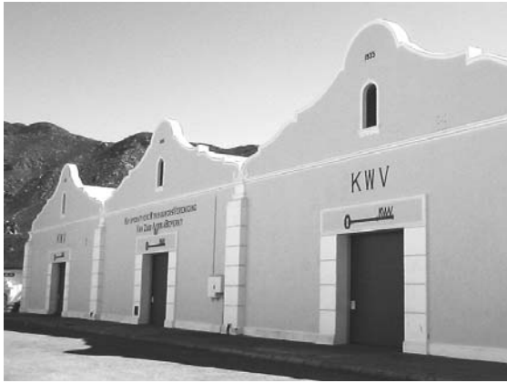
Figure 13: Three 1930s KVV buildings, with Kohler Street in the foreground.
