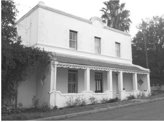
Figure 5: A double-storey, parapeted house on Rawson Street, with simple plaster mouldings and timber verandah detailing.
