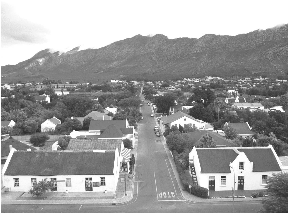
Figure 12: A photograph taken from the clock tower of the Dutch Reformed Church, looking south along Church Street, with Bath Street running from left to right in the foreground. The view is framed by two early-Victorian thatched houses on each corner.
