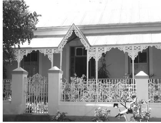
Figure 6: No.39 Joubert Street, with delicate timber verandah detailing and cast iron boundary wall detailing.
