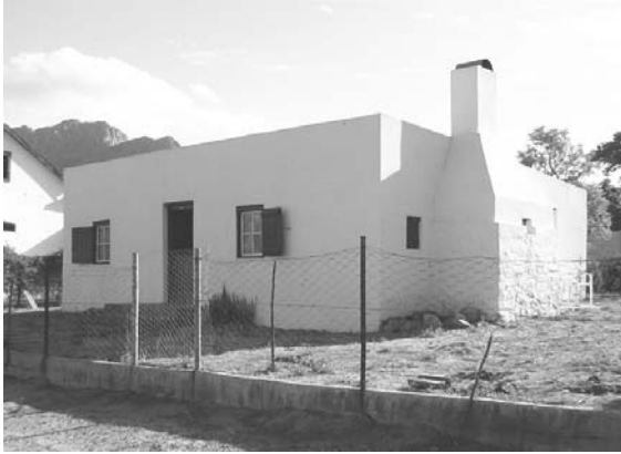
Figure 8: A flat-roofed vernacular cottage on Krom Street in Montagu West
