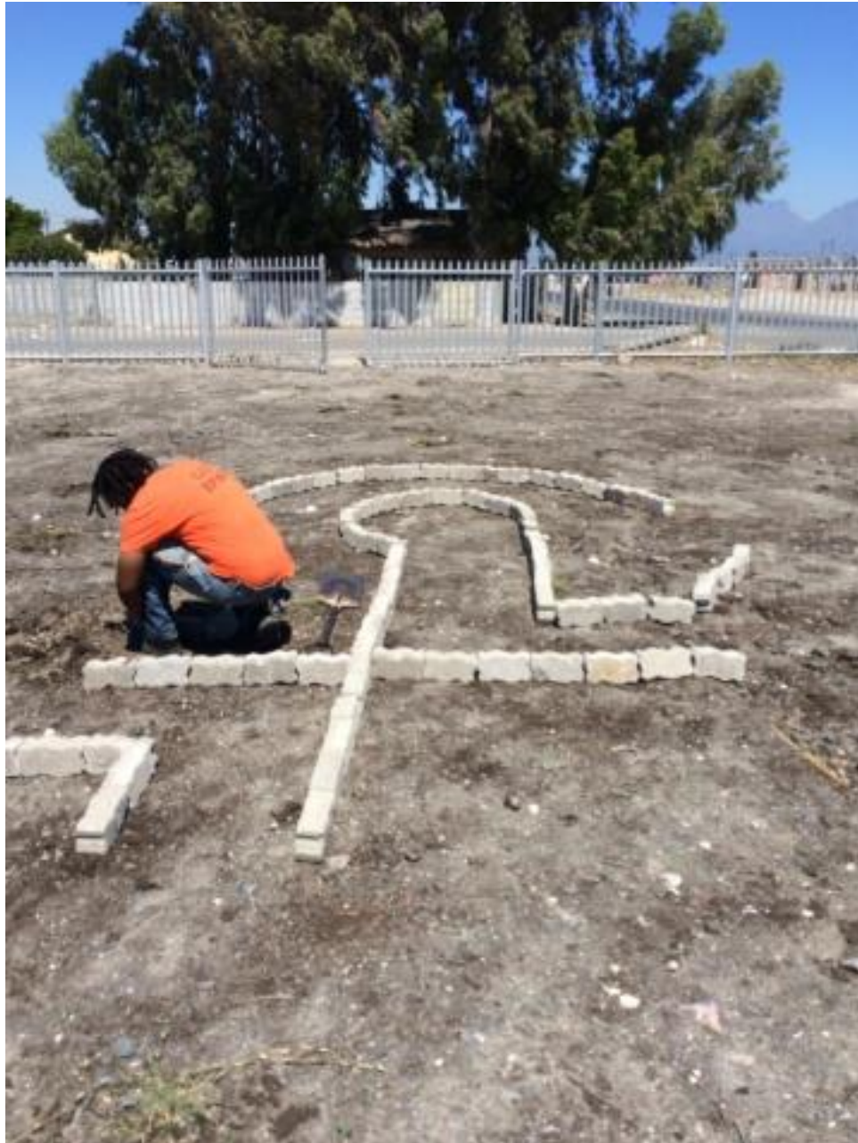
Figure 40: Building the Labyrinth (30 November 2016)
