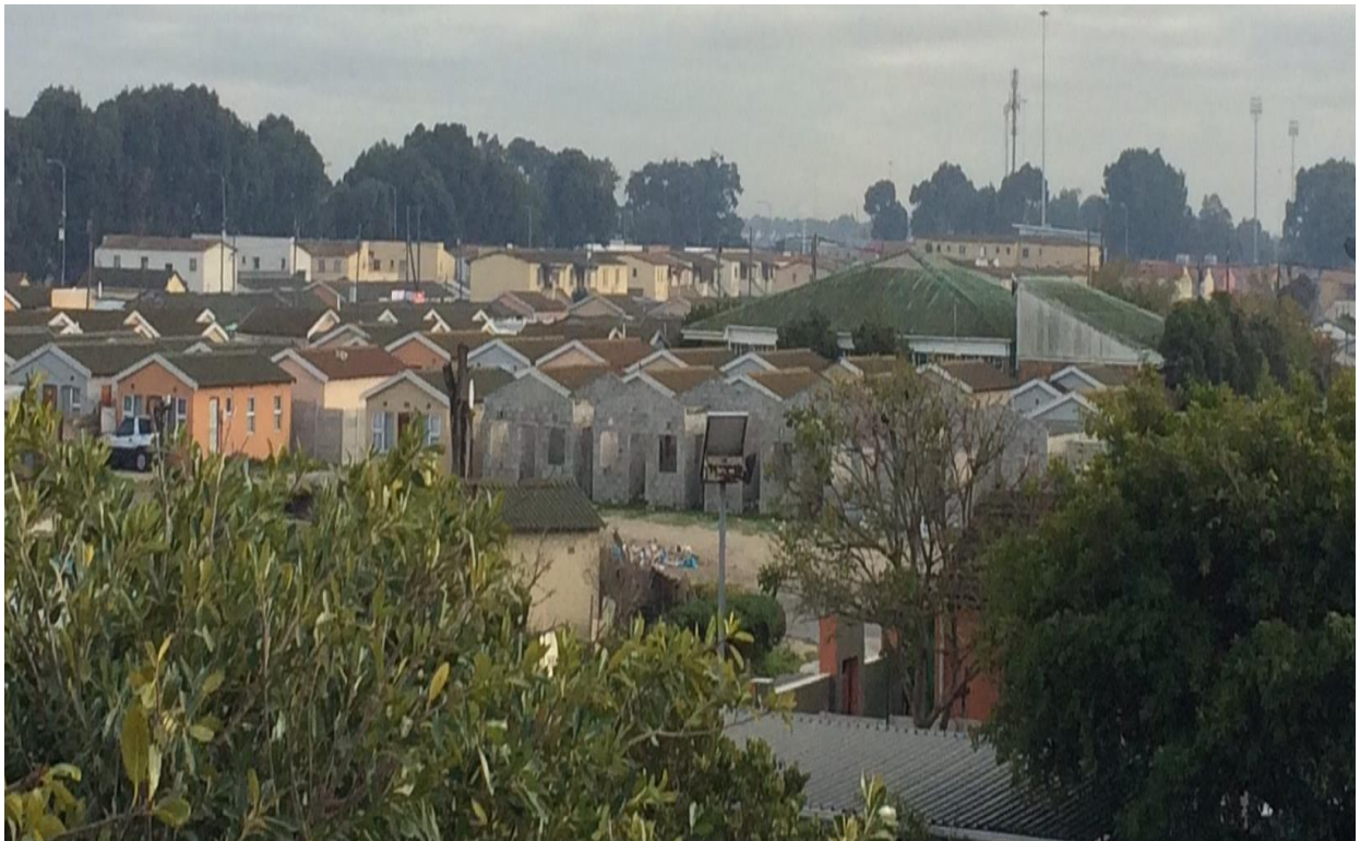
Figure 11: RDP houses in the foreground and new hostel flats in the background (19 July 2017)
