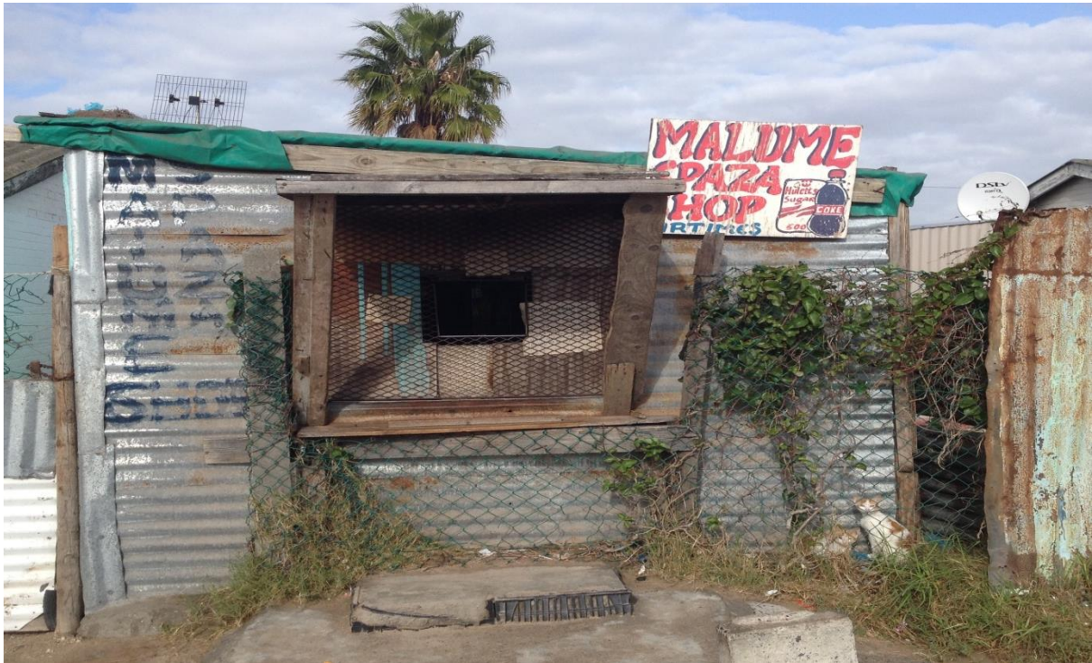
Figure 8: Spaza shop along Miller Road, Nyanga (9 May 2017)
