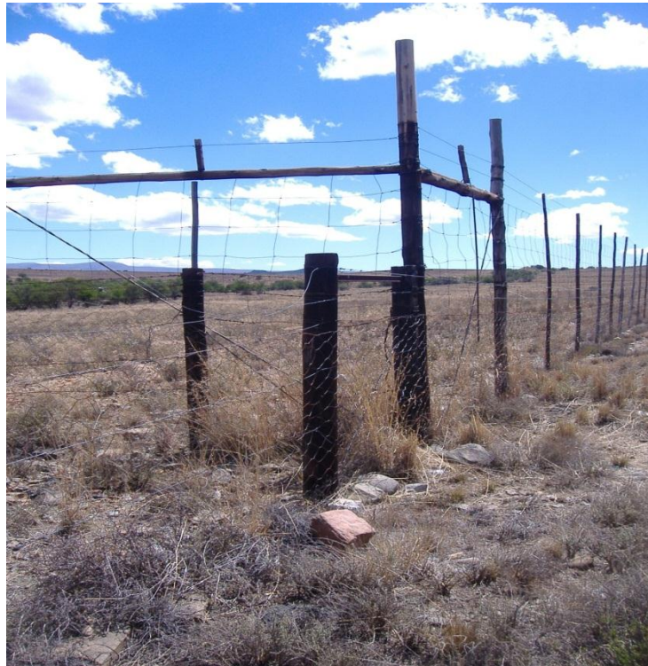
Figure 6: The Bontebok Private Nature Reserve 2.4 metre high game fence next to a conventional short fence of the neighbouring farm
