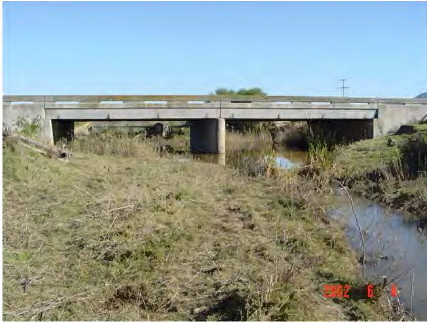
Figure 6.10: Bridge (B5031) across Sand River
