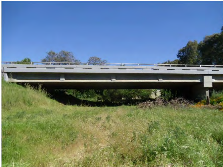
Figure 6.12: Berg River Bridge
