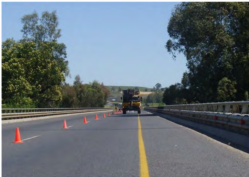
Figure 6.22: Mobile crane and bridge interaction
