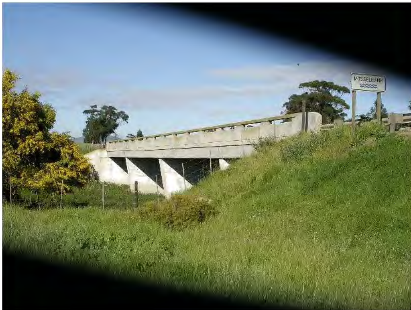
Figure 6.11: Bridge (B5032) across Bot River
