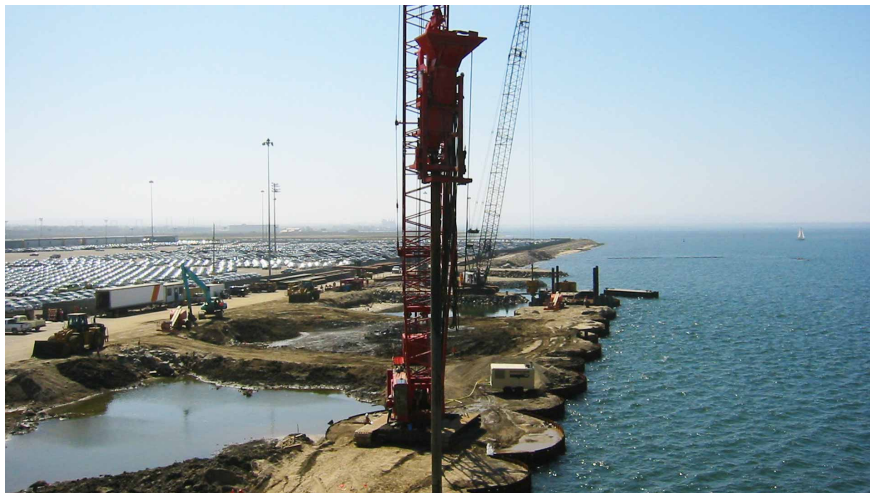
Figure 2.51 – Vibro concrete column crane hung assembly (Menard, 2016a)
