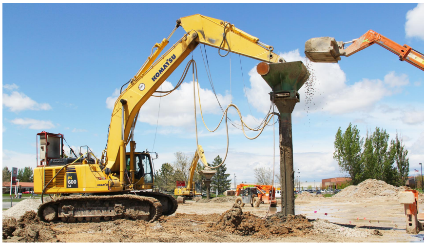
Figure 2.50 – Vibro concrete column installation (Menard, 2016a)
