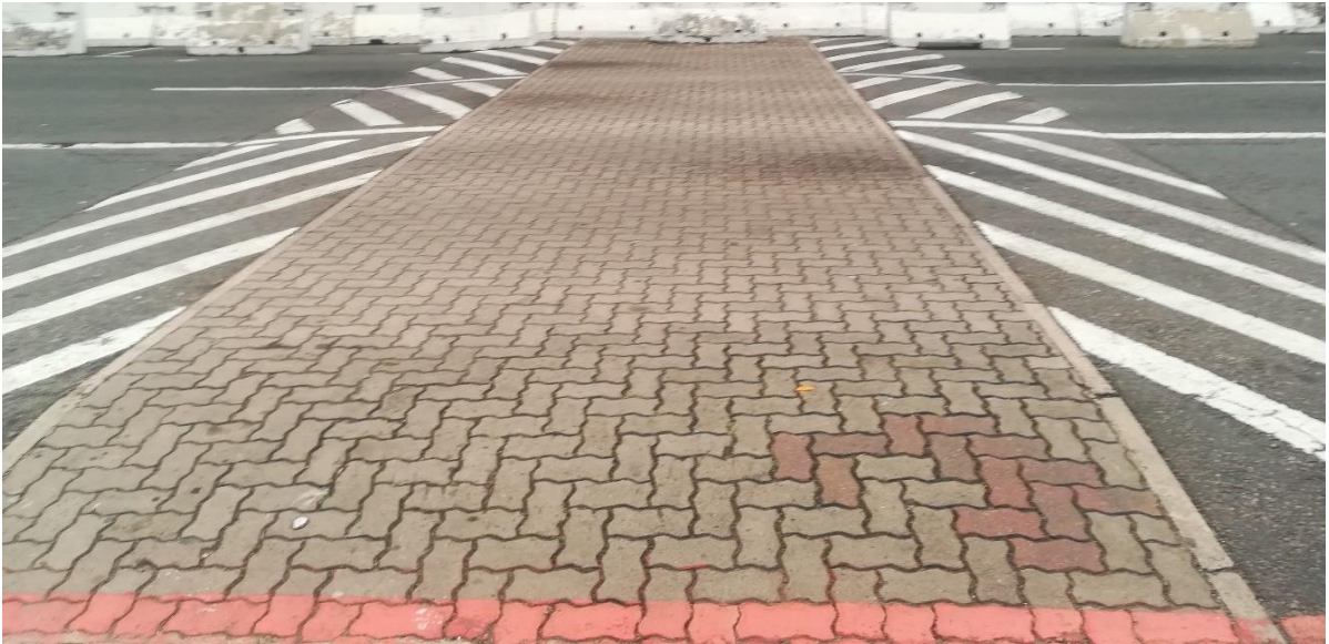
Figure 9: Speed table at Old Fort Road, Durban
