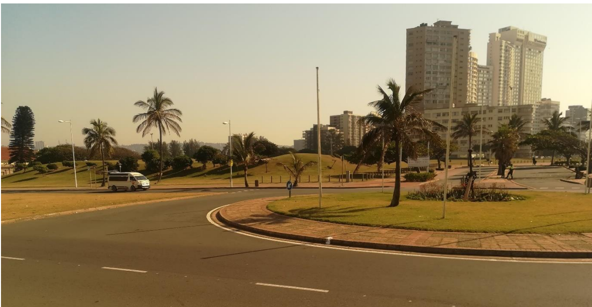
Figure 12: Raised Crosswalk, KE Masinga road, Durban
