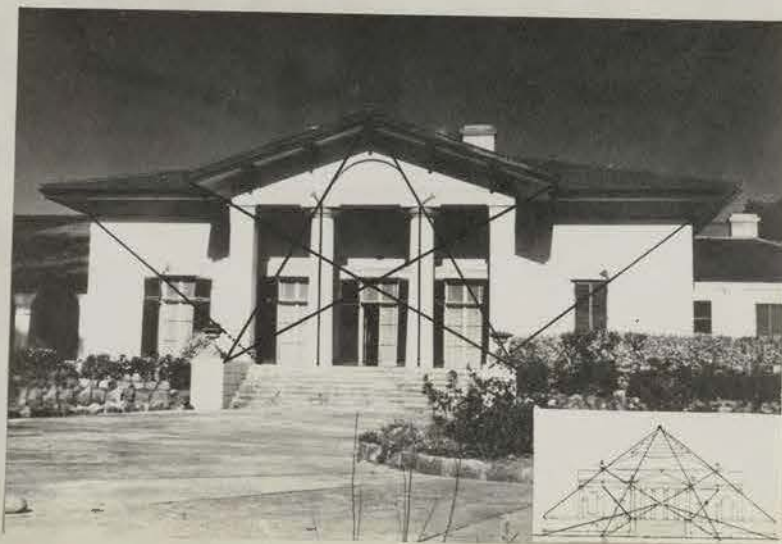
35. 'Belmont', Rondebosch, compared with an interpretation of Palladio's Villa Rotonda. (The distortions in the photograph have been compensated for).
