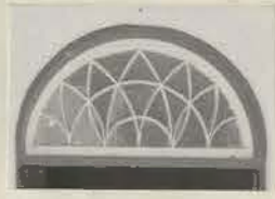
15.A. Geometrically designed fanlight based on intersecting arcs; from George.
