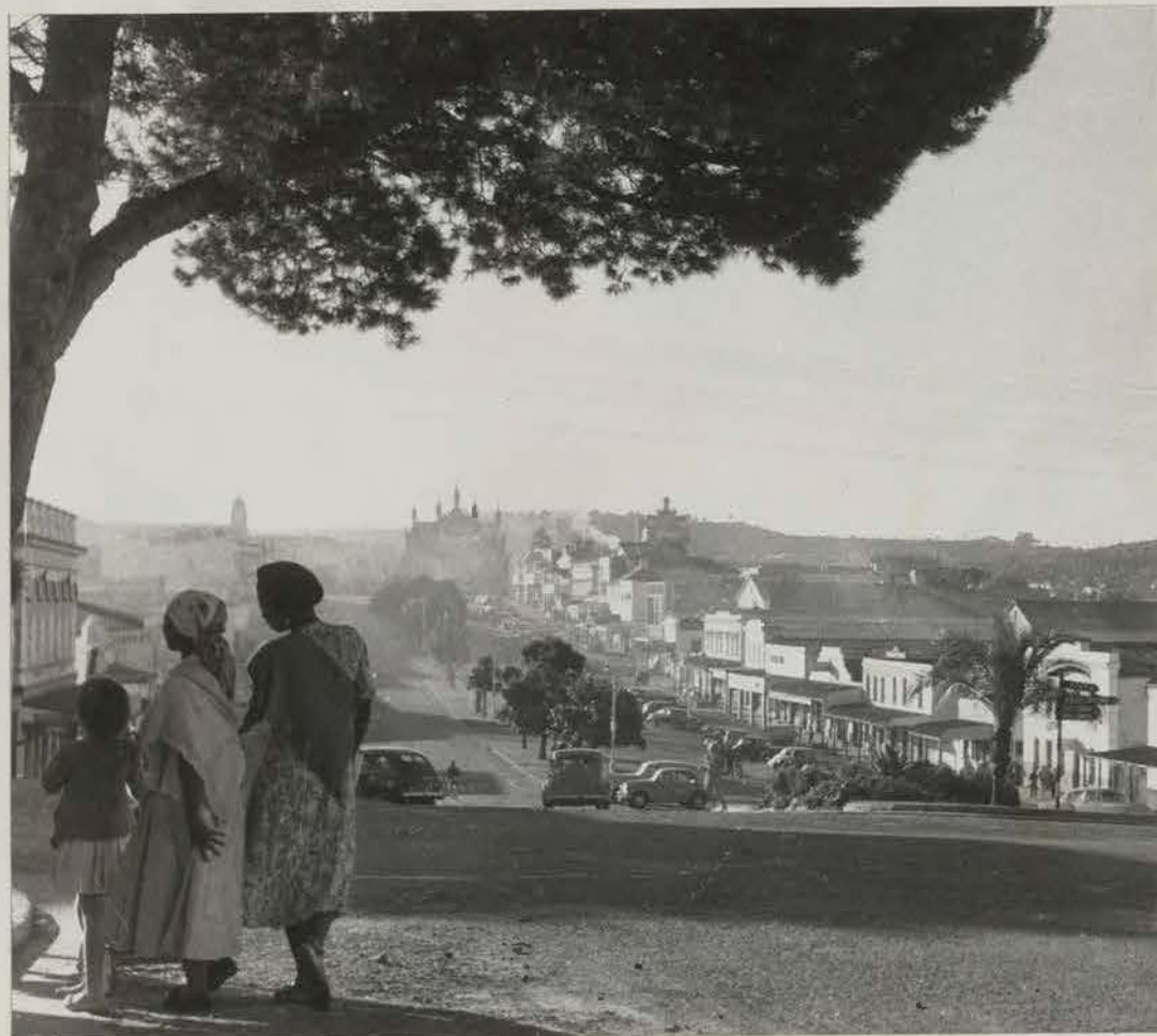
22. View down Bathurst Street, Grahamstown, with the Settler Church closing the vista; from Beaufort Street.
