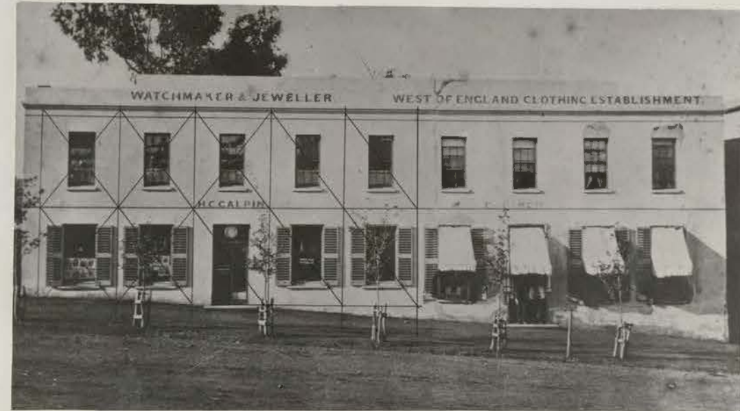
33. Bay designing in Bathurst Street, Grahamstown.
