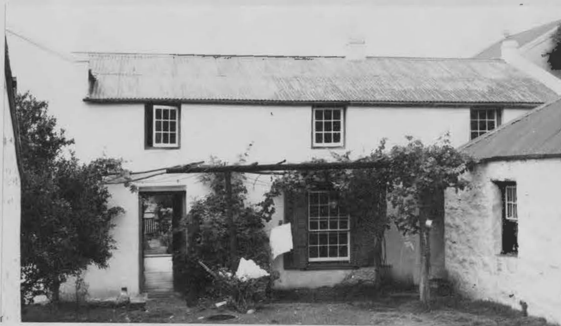
25. House on the Keerbooms River, Cape. ± 1830.
