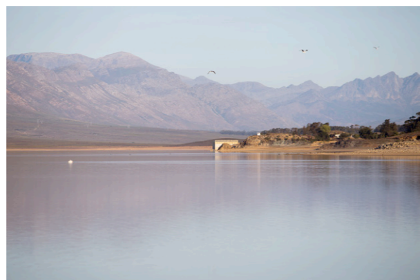
FIGURE 43. VOELVLEI DAM NEAR GOUDA SOURCE: ASHRAF HENDRICKS
