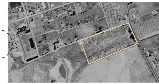
FIGURE 60. OKUULOF IN 1965- ALL DWELLINGS AND THE CHURCH ARE DEMOLISHED
