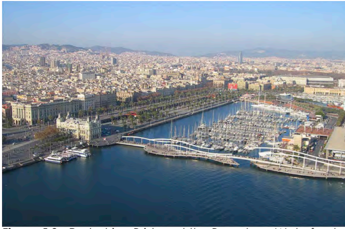
Figure 5.2 - Pedestrian Bridge at the Barcelona Waterfront. (Source: Yeh, 2015).
