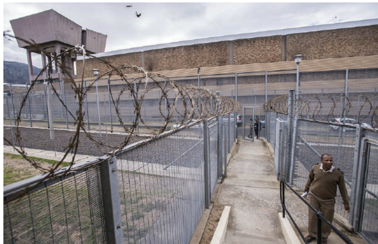
figure 3: threshold into current visiting facilities in prison blocks
