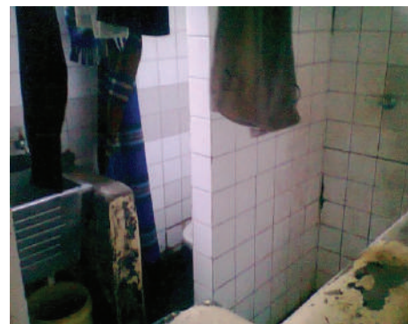
figure 32: toilets within communal cells
