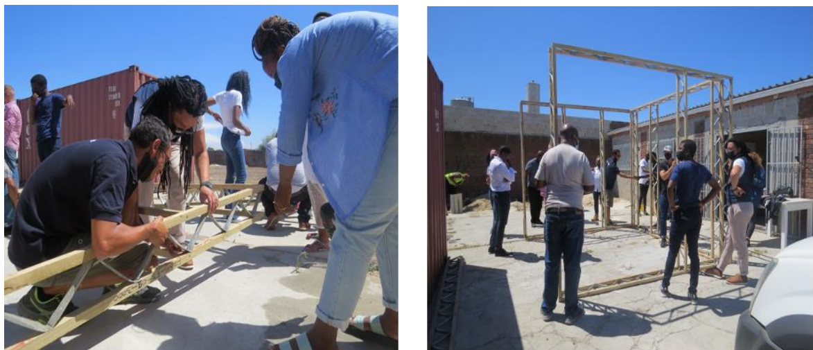
Figure 8: Example of sandbag house with eco-beam (timber) frame walls
