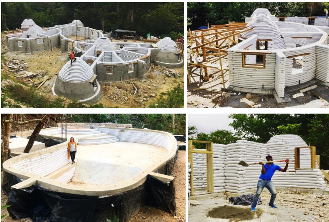
Figure 6: Sandbag house construction including a swimming pool
