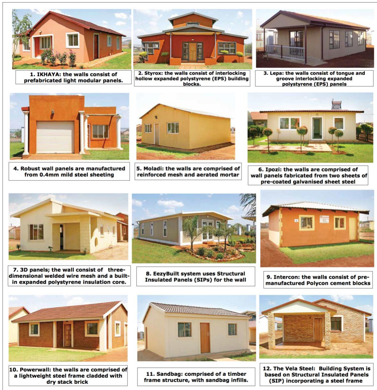
Figure 4: ABTs at Eric Molobi Housing Innovation Hub (National Home Builder's Registration Council, 2020)
