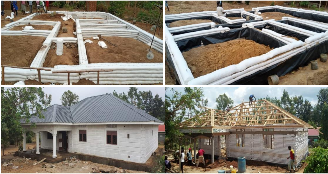
Figure 7: Example of the construction of a super adobe sandbag house.
