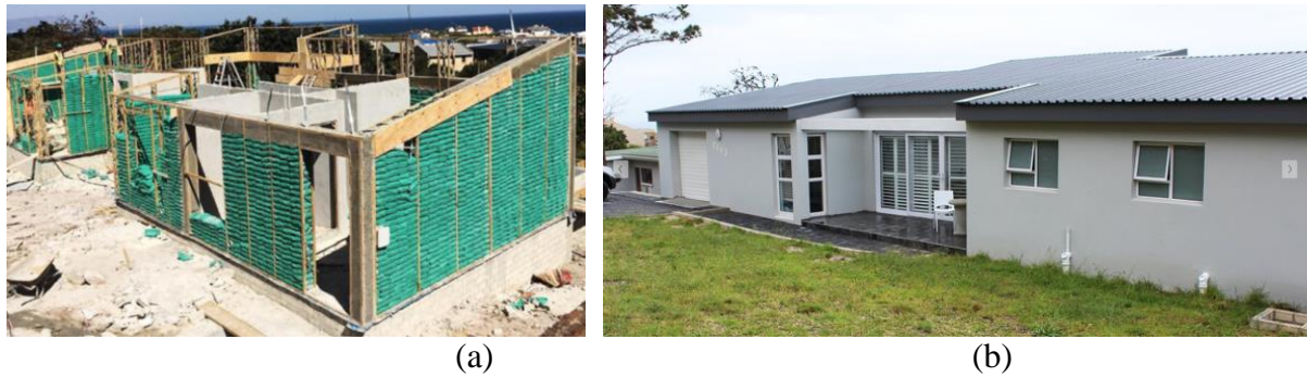
Figure 11: (a) SBT house under construction; (b) SBT house post-construction
