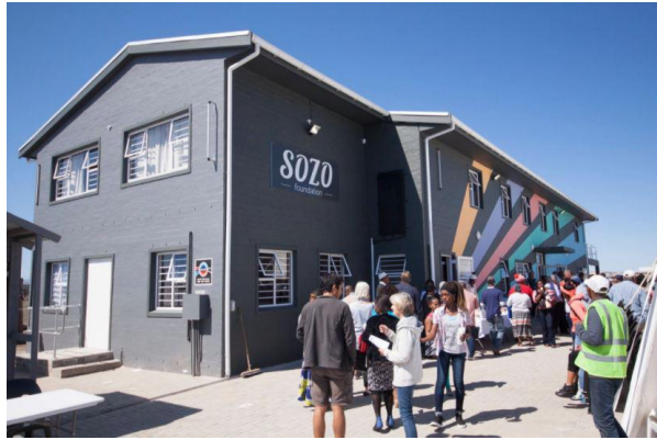
Figure 4-3: The vibrant looking Sozo Building located in the heart of Vrygrond.
