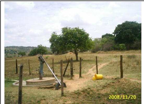
Deep well servicing Shumba clinic
