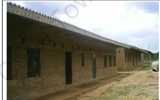
New classroom block being constructed by new responsible authority at Mtanhaurwa Primary School
