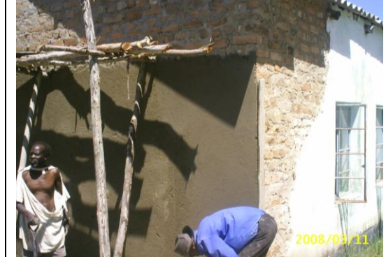
Repair of classroom at Kanongovere Primary School undertaken by parents from community contributions and donated local labour
