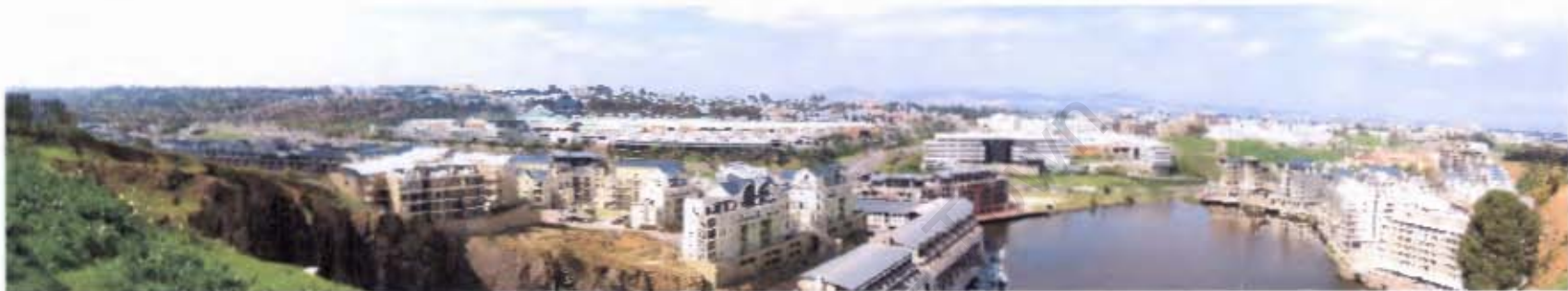
Figure 4.6: Tyger Waterfront and Tygervalley Centre in background, 2006
