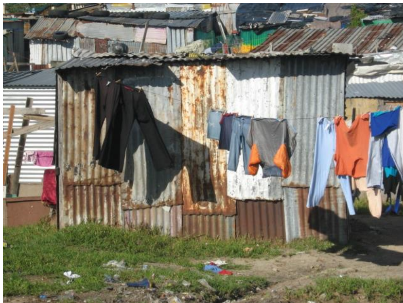
Figure 5.1. A Shack on an un-serviced site in Khayelitsha Site C
