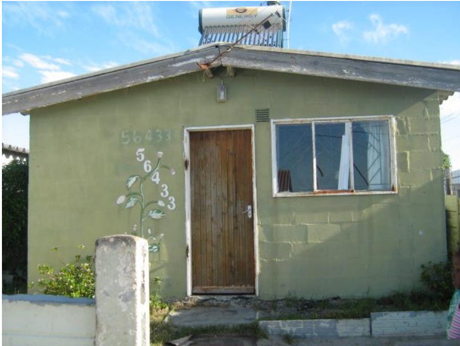
Figure 5.2. A house obtained through a housing subsidy in Kuyasa
