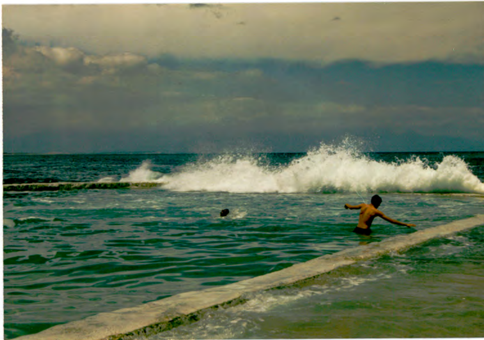
Plate 1.1 : Overtopping at St James tidal pool
