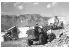
Demolition of District Six, photo by Stan Abrahams, late 1960s District Six Museum
