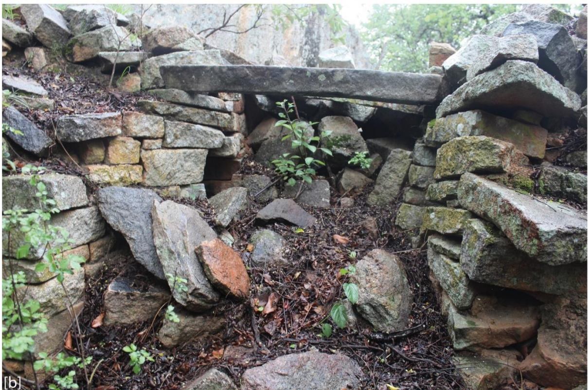
Figure 7.2: [a] part of the dry-stone walling at Chumnungwa (including the conical buttress) built on top of protruding flat granite outcrops, [b] One of the squared entrances with a dolerite stone slab used by stonemasons as lintels for buttressing the squared entrance at Chumnungwa.
