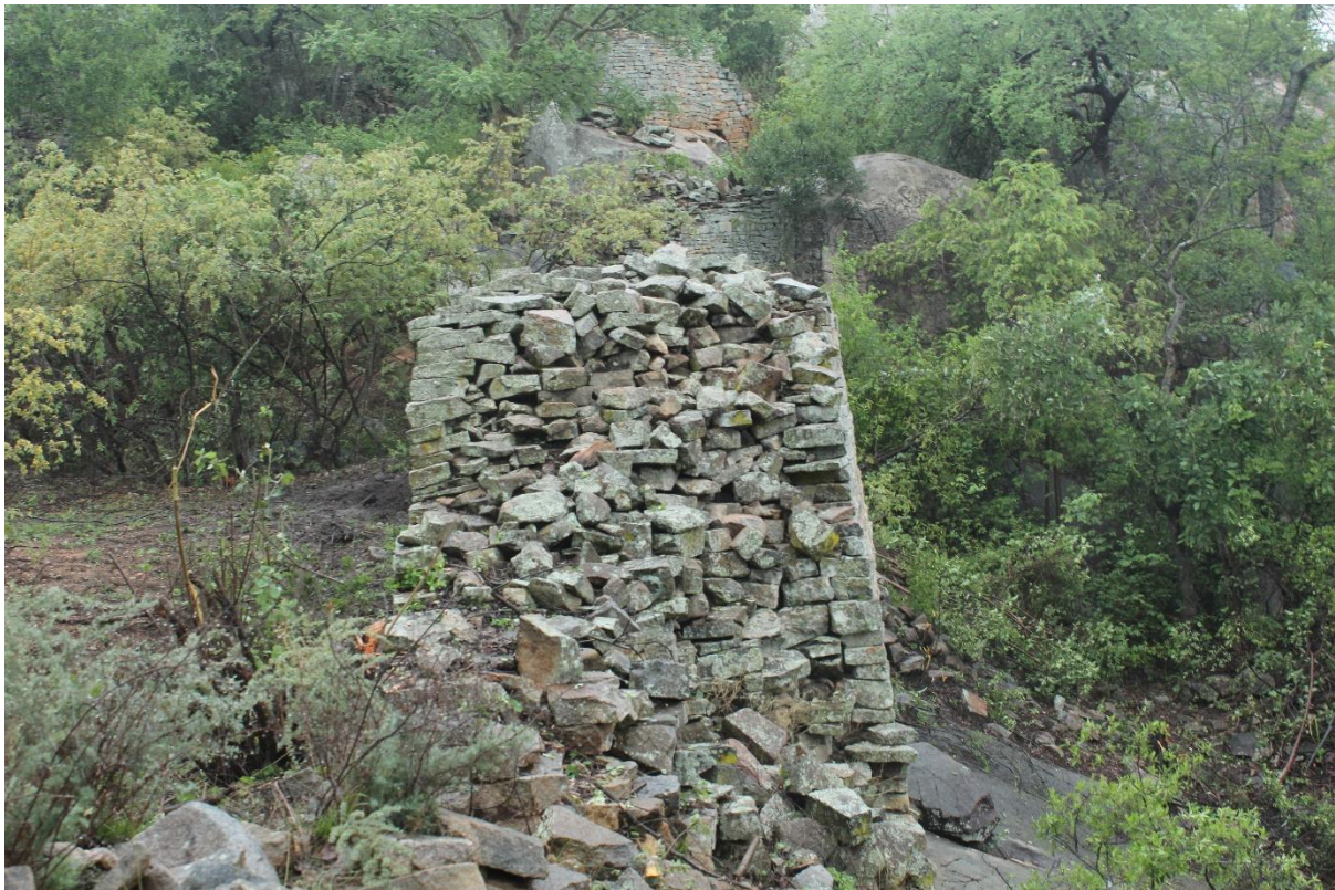
Figure 7.7: A cross-section showing the inner (undressed blocks) and outer (dressed blocks) of Wall 1d.
