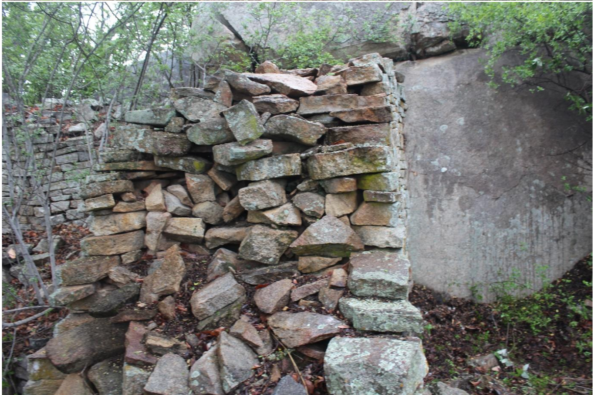
Walls 6b, and 6c
