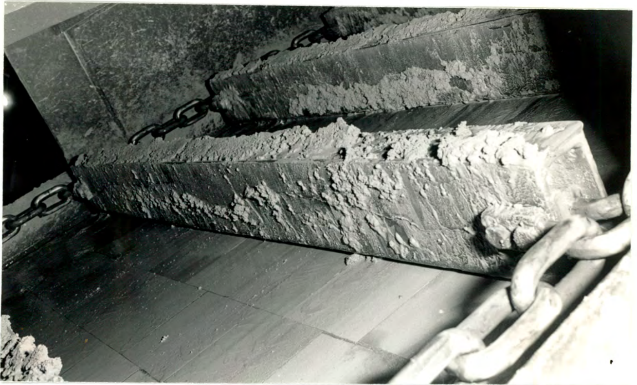
Figure 1.3 Return side of the drainage deck of a submerged scraper conveyor. Flights are suspended between two parallel running chains. Flights are seen moving over a surface lined with alumina tiles.
