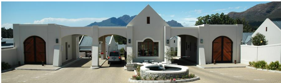
Figure 20: Security entrance of La Clémence Retirement Village. Note the gable doors and water feature. (Photograph Havenga 2018)
