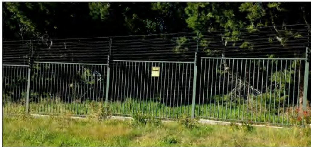
Figure 2.8. Photograph of the 2.5m high Steenberg electric security fence. It includes upright metal bars with 12 electrified wire strands on the exterior surface, and 24 electrified strands lining the interior surface of the fence.
