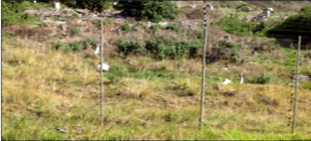
Figure 2.7. Photograph of the Zwaanswyk electric fence from within the residential area looking towards TMNP. The 2.4m high fence has 15 electrified strands (80 000V), with a four-strand overhang. The fence also includes fine wire mesh to prevent baboons from forcing their way through the strands.
