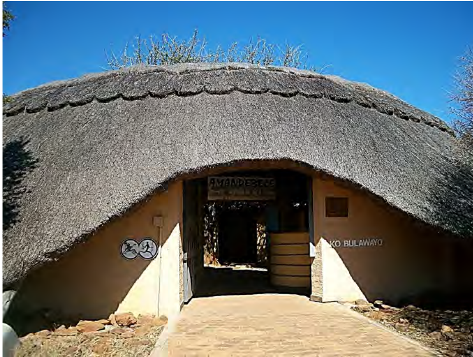
Figure 14: The Interpretive Centre at the Main entrance to the Old Bulawayo historical site
