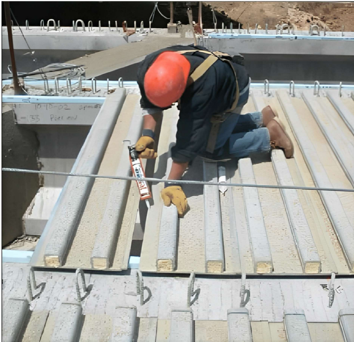
Figure 2-7: Fibre cement boards used a non-participating formwork (Malla et al., 2007)
