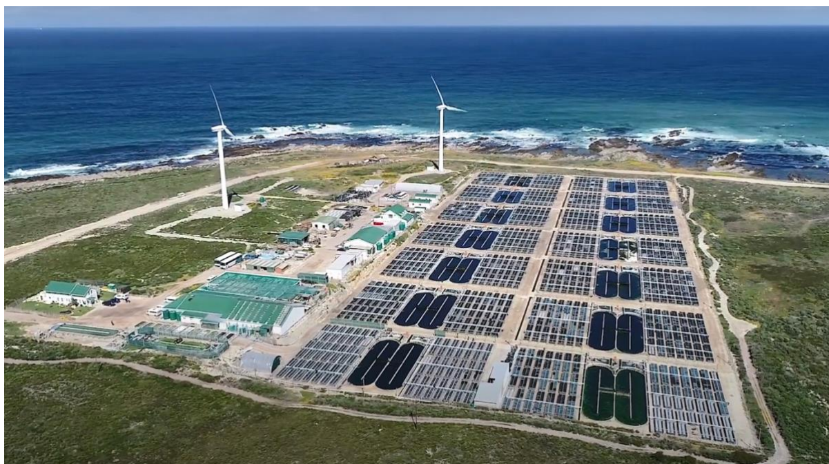
Fig. 1.2. A commercial recirculating land-based abalone- Ulva integrated multi-trophic aquaculture system in Buffeljags, South Africa. Here, Ulva lacunculata is cultivated in 28 paddle raceways (approximate surface area of 300m 2 each) using effluent of Haliotis midae , which are grown in more than 1 100 tanks (8.5m 3 volume each) resembling cells adjacent to the Ulva ponds. The Ulva provides both feed and bioremediation for the abalone. Source: www.vikingaquaculture.co.za
