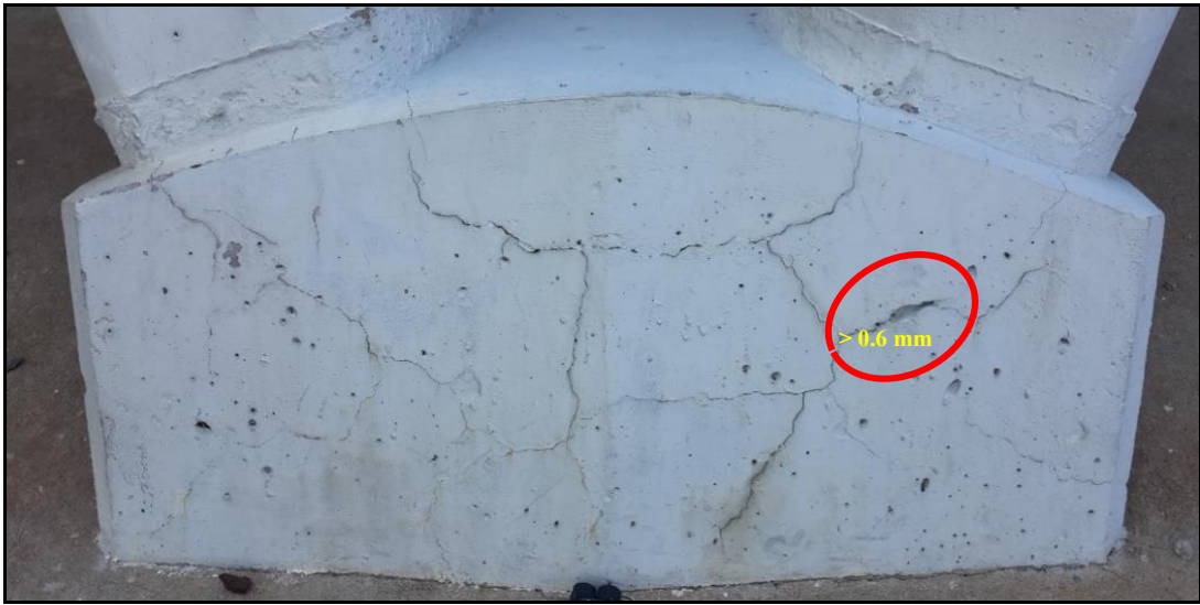
Figure 34: Pedestal 03 – Front view
