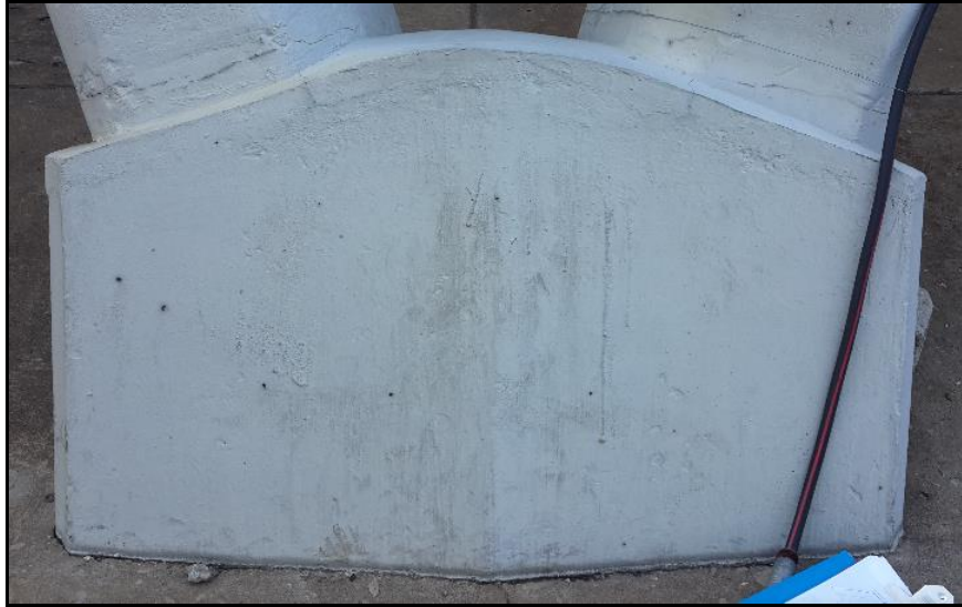
Figure 32: Pedestal 01 – Front view
