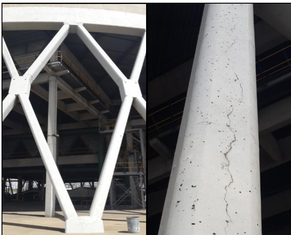
Figure 36: Lower Column of Pedestal 18
