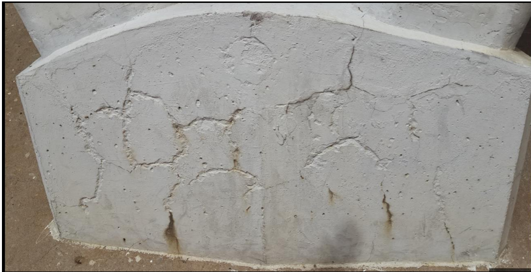
Figure 35: Pedestal 28 – Front view
