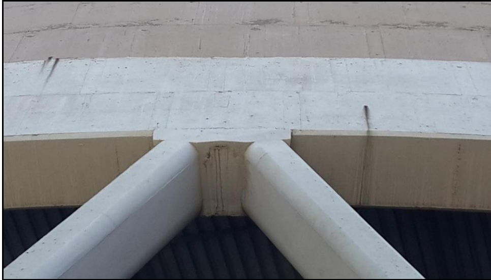
Figure 37: Bottom of the dry cooling tower shell
