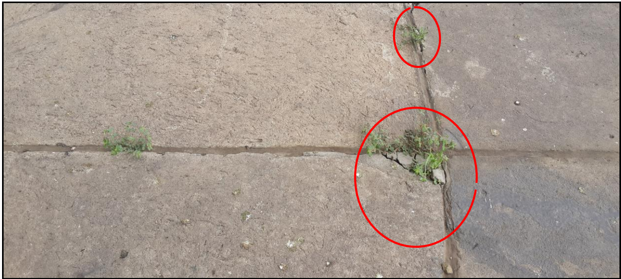
Figure 38: Expansion Joints (Floor)
