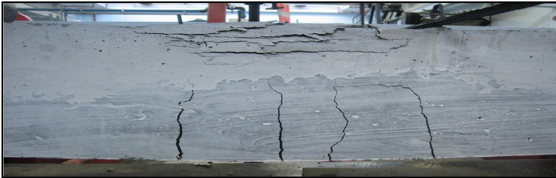
Figure 6.8b: Crack pattern on Beam 3 during failure
