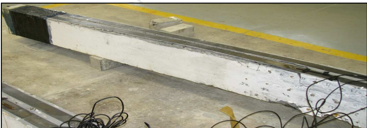
Figure 6.8c: Crack pattern on Beam 2 during failure
