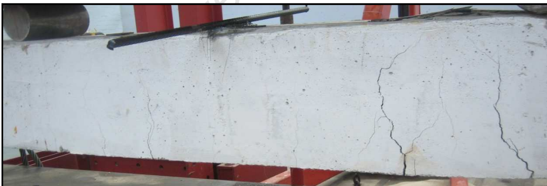
Figure 6.8a: Crack pattern on Beam 1 during failure
