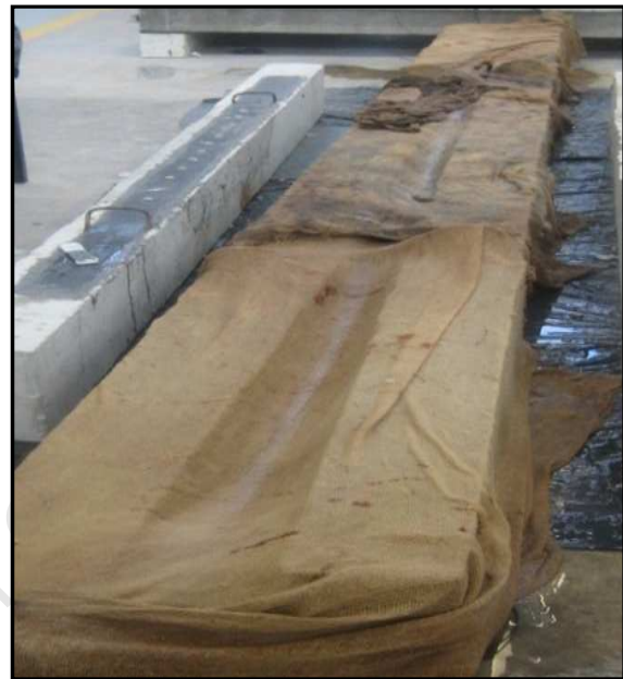
Figure 3.5: Curing with a Hessian cloth
