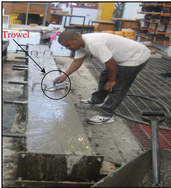
Figure 3.4: Concrete after casting
