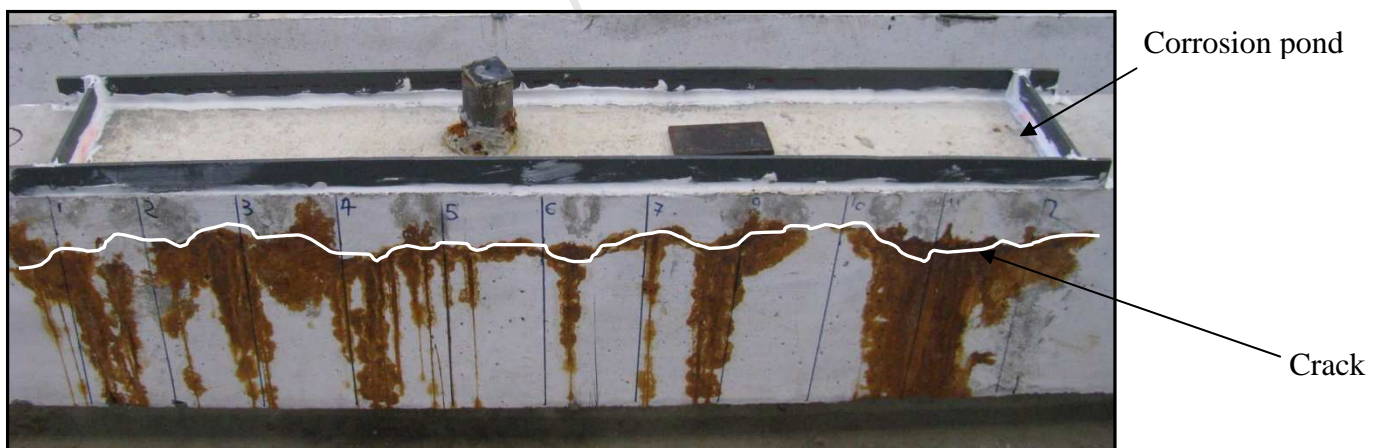
Figure 4.2a: Crack pattern for Beam 2.
