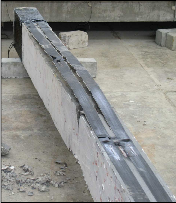
Figure 6.8d: Crack pattern on Beam 4 during failure
