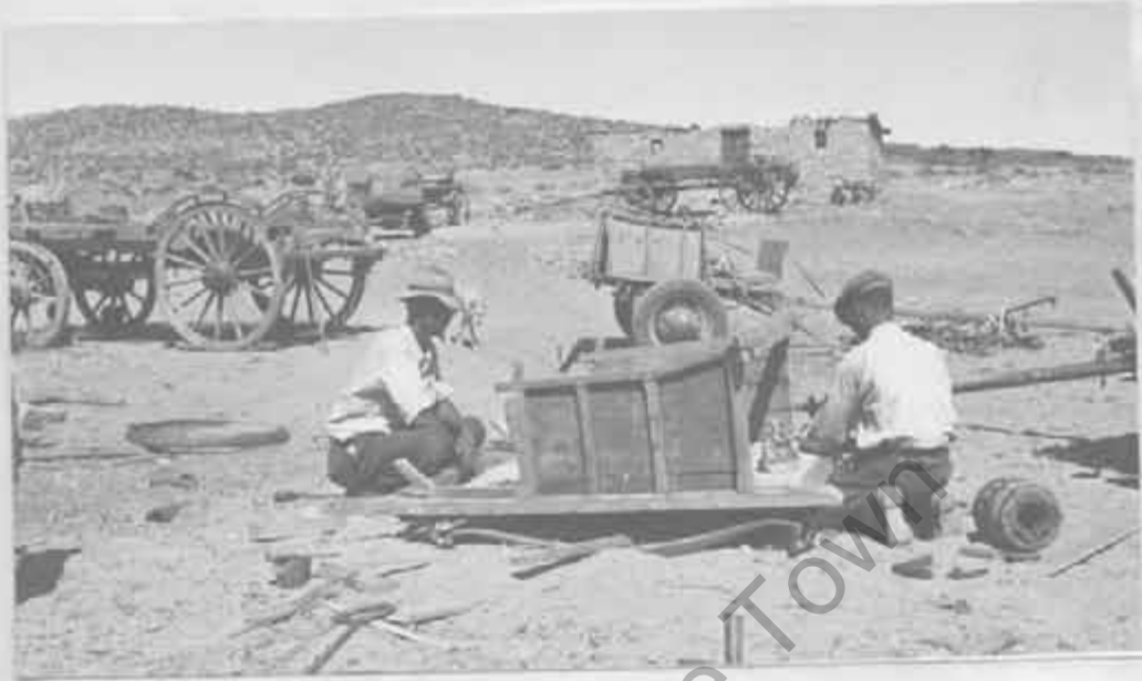
4. REPAIRING WAGONS IN A HAMLET
