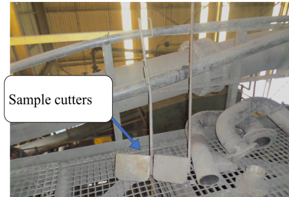
Figure 4-4: Picture showing the sample cutters used for cutting samples
