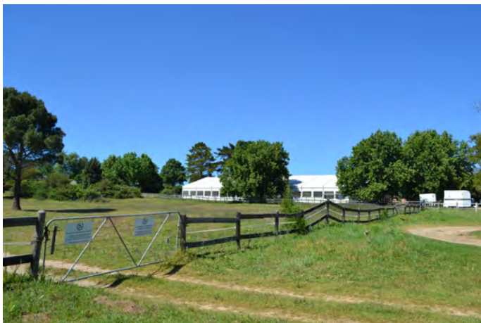
Image 3 Infrastructure on Erf 142 used for equine maintenance and riding lessons. Infrastructure is catered to disabled individuals needs.
