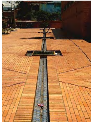
Figure 64 Nueva Santa Fe housing complex stormwater paving detail by Rogelio Salmona
