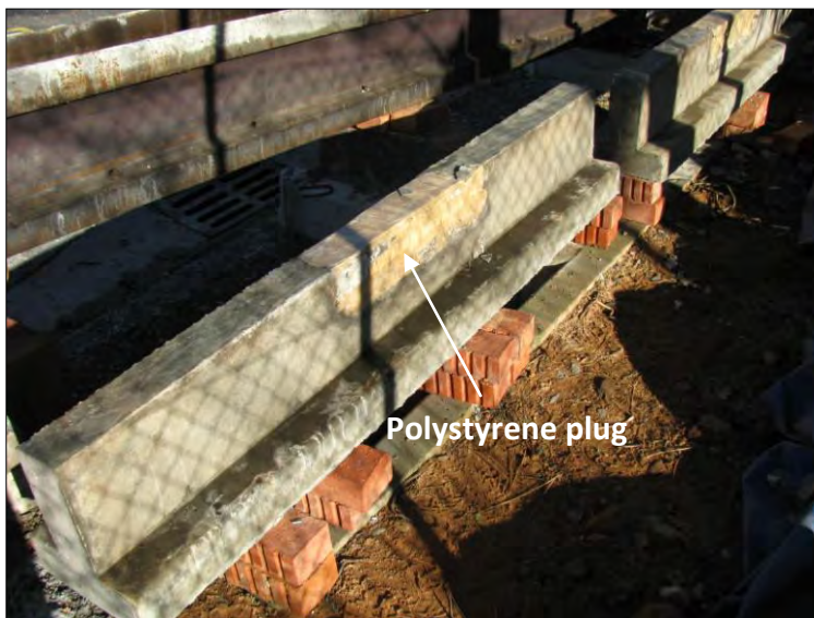
Figure 43: Demoulded beam with polystyrene plug
