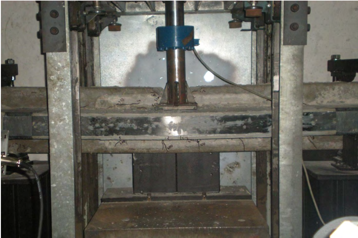
Figure B10: Damage observed after consecutive drop tests conducted on beam R-80
