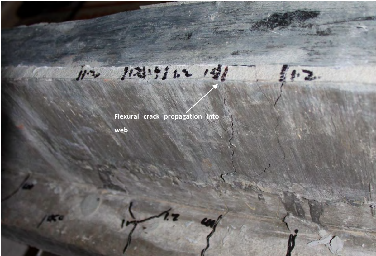
Figure B19: Flexural crack propagation (beam R-160)
