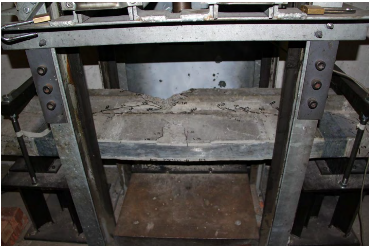
Figure B17: Damage observed after consecutive drop tests conducted on beam R-160
