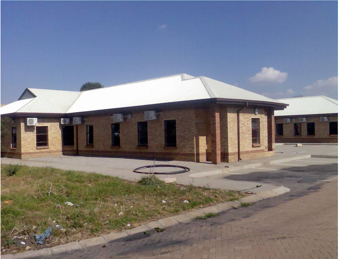
Appendix 2 Photograph: Admin block - completed in 2006 but not handed over due to absence of electricity
