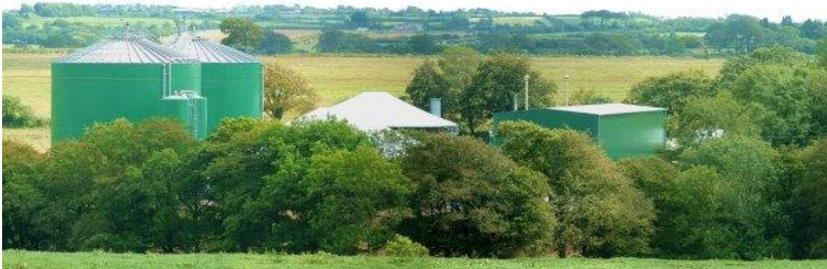
Figure 2-10: Holsworthy Biogas Plant in UK (Source: Pace 2013)
