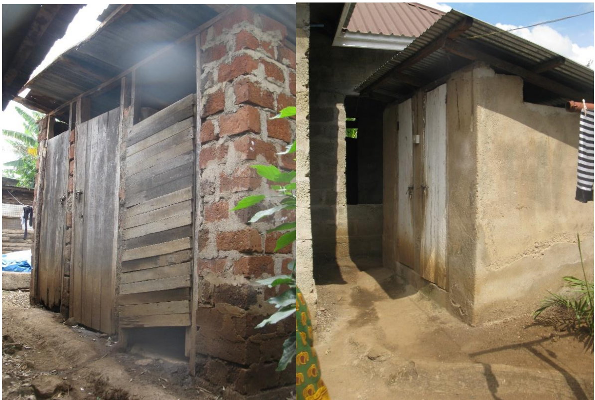
Figure 8. 11: Some of the burnt brick and cement block structures in Baraa Source: Fieldwork, 2014
