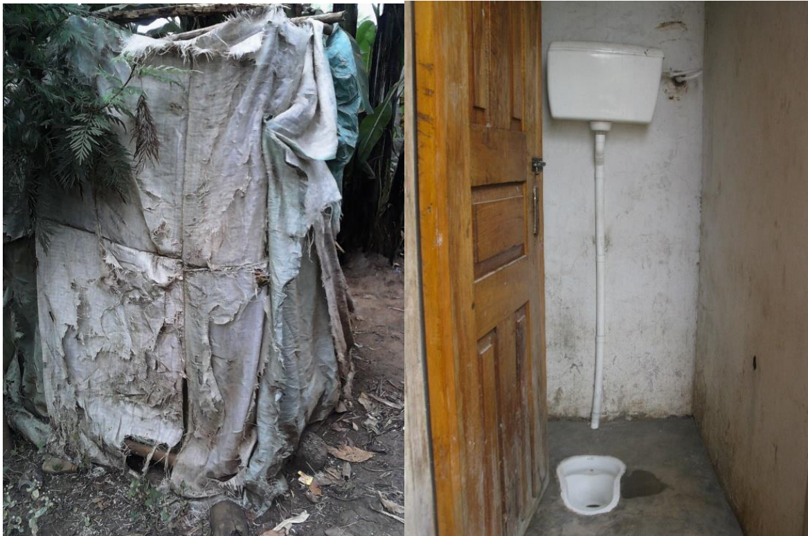
Figure 8. 8: Toilet facilities in Sombetini ward: Traditional latrine (left) and a flush toilet (right). Source: Fieldwork, 2014
