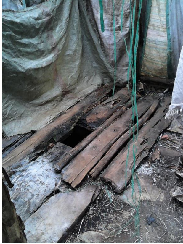
Figure 8. 15: Super structure made of sacks as walls, and raw timber for the base in Sombetini. Source: Fieldwork, 2014
