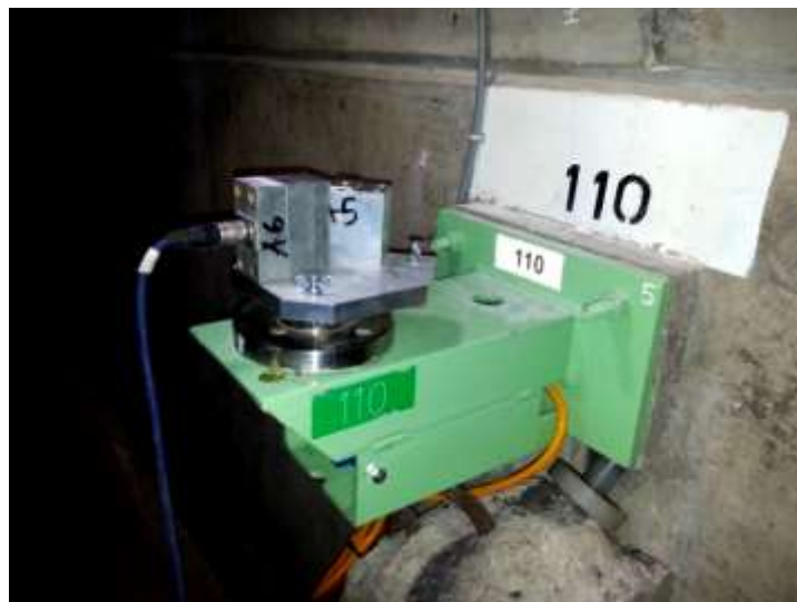
Figure 30: Roving and permanent accelerometers
