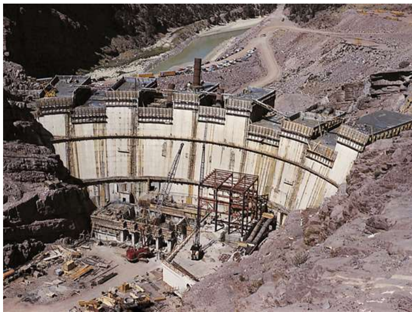
Figure 4: Flaming Gorge dam construction in 1962 (USBR, 2016)
