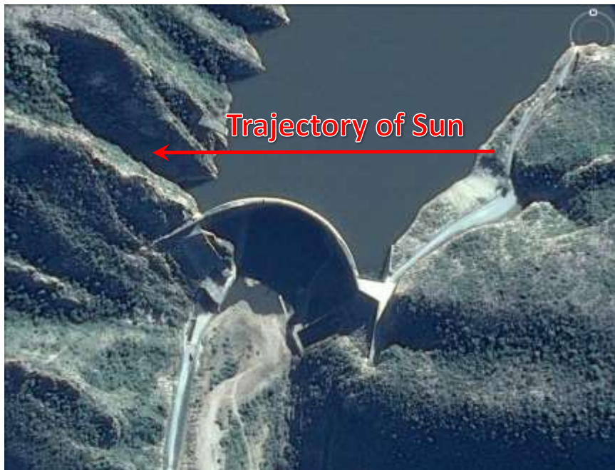
Figure 32: Trajectory of the Sun across the dam wall
