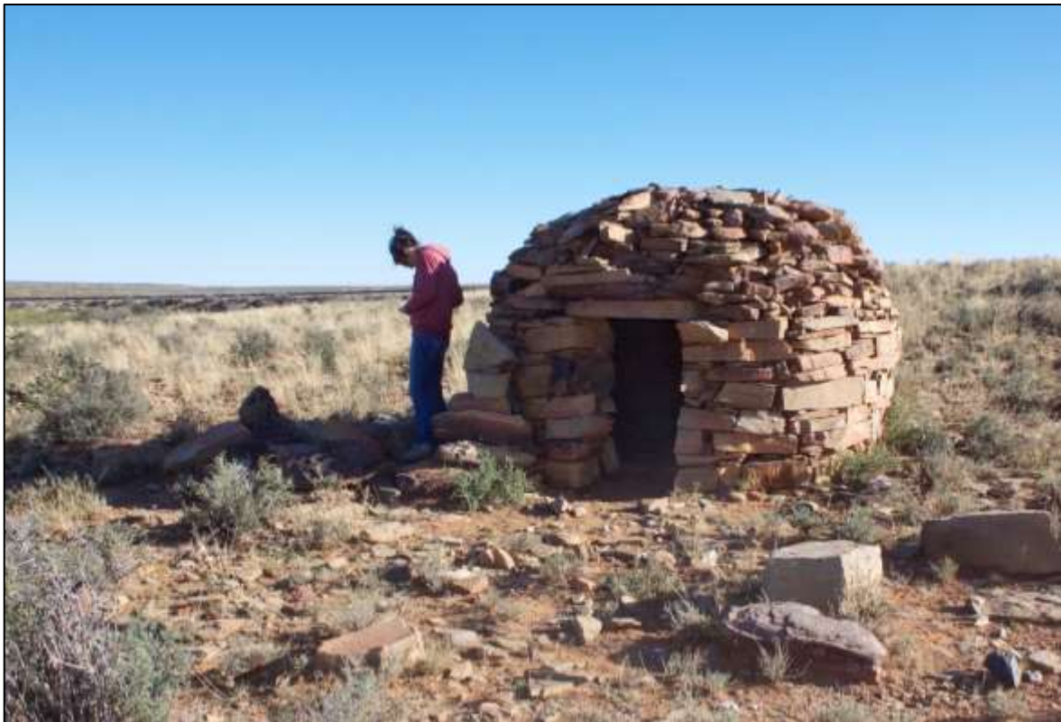
Figure 5 Small corbelled building on Droogeputs Farm located on the R63 between Carnarvon and Williston.
