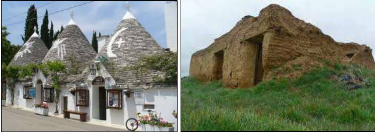
Figure 16 Images of Left: Trulli of Puglia in southern Italy, right: corbelled dome in Tierra de Campos, Spain (Kramer, 2012: 7).
