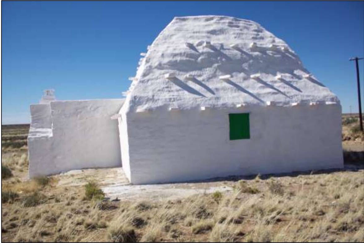
Figure 4 Rectangular based corbelled building with white plastered walls on Arbeidersfontein farm located on the R63 between Williston and Carnarvon.
