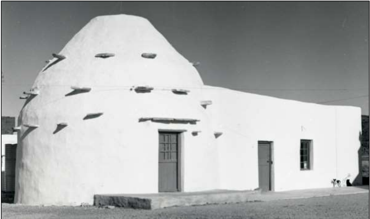
Figure 2 Photograph of corbelled building on Grootfontein which was declared a national monument in 1968. (Walton, 1960)
