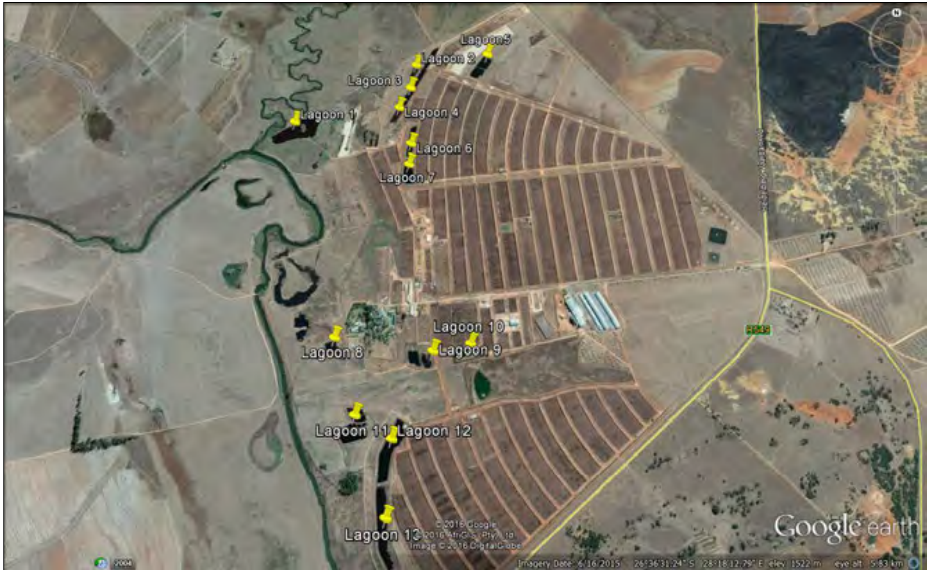
Figure 13: Effluent lagoons on the Study Site.
