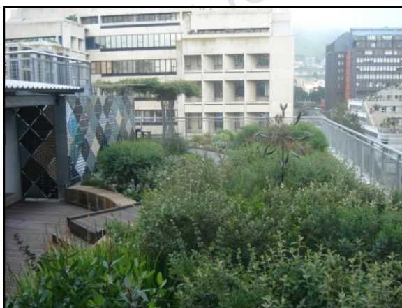
Figure 2.6: Intensive green roof, City of Cape Town CBD
