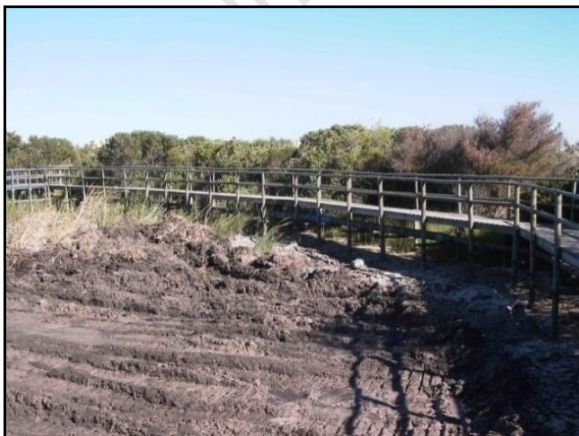
Figure 5.9: Treated effluent discharges beneath Cell 1 walkway
