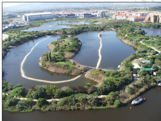
Figure 5.1: Constructed Wetland, Century City, Cape Town
