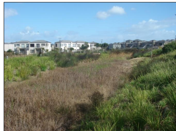
Figure 5.5: Extended detention pond, Century City, Cape Town
