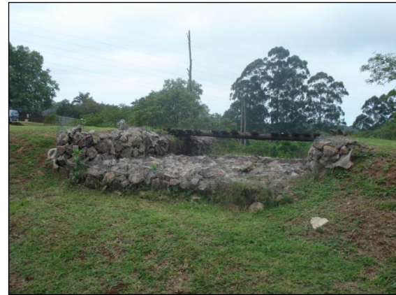
Figure 5.4: Detention pond emergency overflow structure, New Heritage Market, Hillcrest
