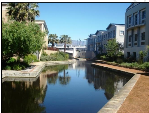
Figure 4.11: Canal ‘meandering’ through eastern office park complex
