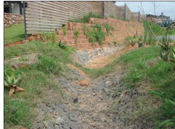
Figure 4.10: Gabion-lined dry swale, Hawaan Estate, Umhlanga
