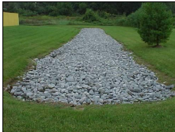
Figure 2.9: Infiltration trench between residential properties
