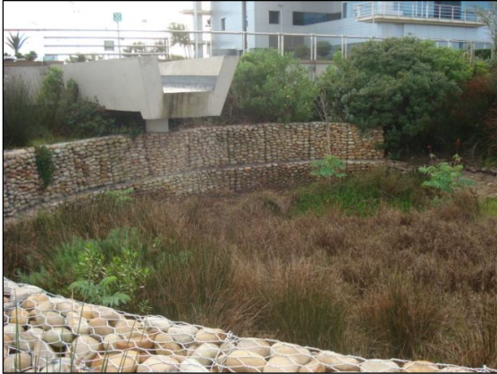
Figure 5.6: Infiltration basin, Century City, Cape Town
