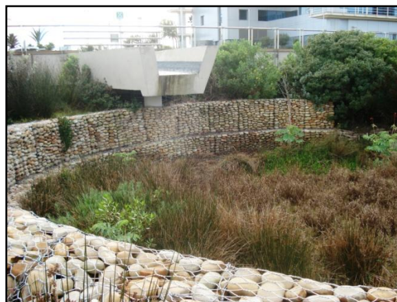
Figure 4.10: Infiltration basin draining a commercial car parking-lot
