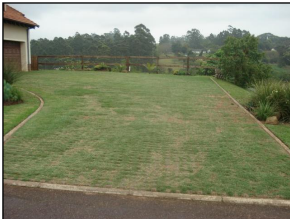
Figure 2.10: Concrete grass block permeable pavement, eThekweni
