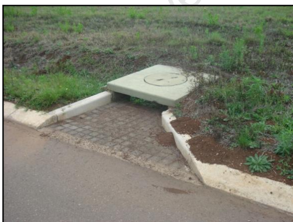
Figure 2.15: Kerb inlet structure directing stormwater runoff into vegetated swale, eThekweni
