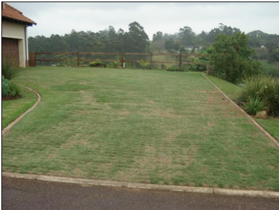
Figure 4.8: Modular pavement system planted with grass, Clifton Hill Estate, Hillcrest
