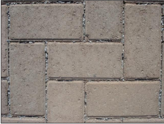
Figure 4.5: Permeable concrete block pavers with open joints and slotted ends filled with pea-sized gravel
