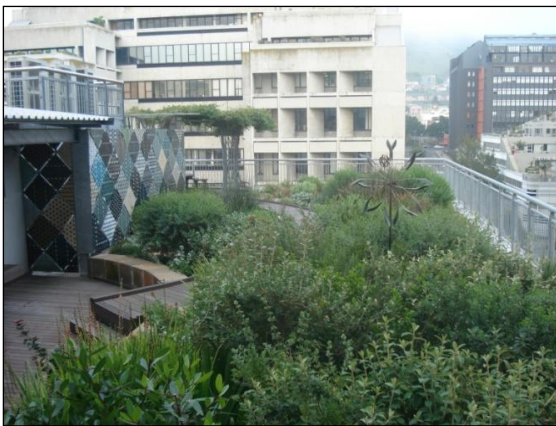
Figure 3.3: Intensive green roof, Department of Environmental Affairs and Development Planning, Cape Town
