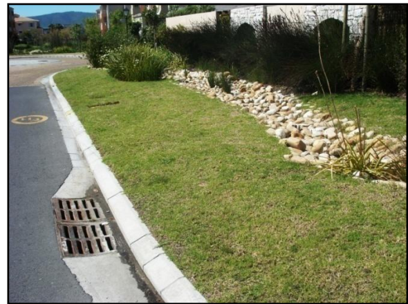
Figure 5.2: Roadside kerb and cast iron catchpit superseding swale
