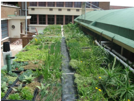
Figure 3.1: eThekweni Green Roof Pilot Project, Durban CBD
