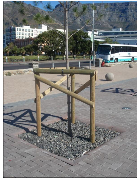
Figure 4.2: Bio-retention rut filled with a coarse aggregate and planted with a tree, Grand Parade, Cape Town
