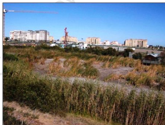
Figure 4.18: Cell 2 during the wetland's construction phase
