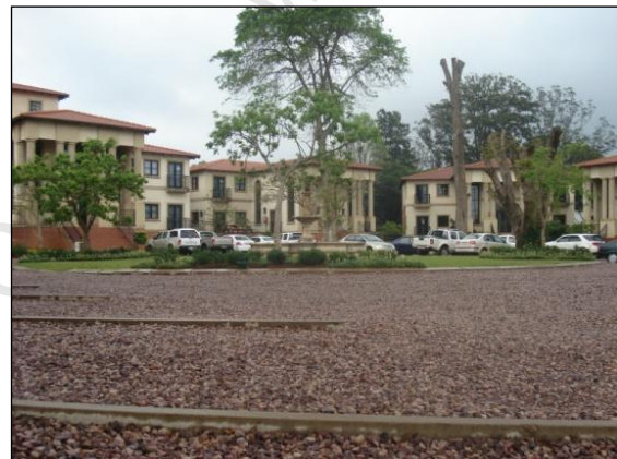
Figure 4.7: Gravel pavement system, Bishops Court Office Park, Hillcrest
