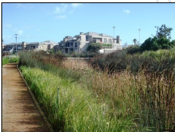
Figure 4.9: Bio-retention corridor at the foot of an infiltration basin
