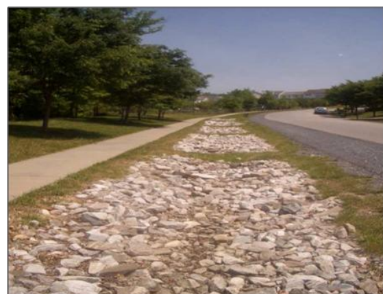
Figure 4.4: Infiltration trench system adjacent to a highway
