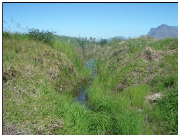
Figure 4.14: Deep grassed ‘wet’ swale
