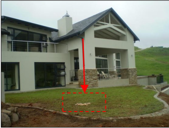
Figure 3.4: Groundwater recharge of runoff from a single residential dwelling, Cotswold Downs Estate, Hillcrest
