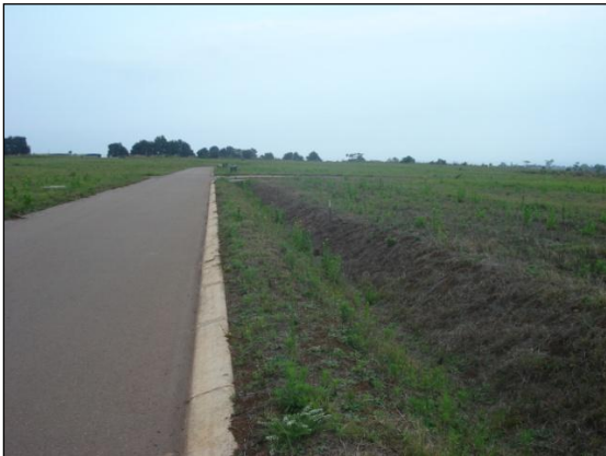
Figure 4.9: Roadside swale, Cotswold Downs Golf Estate, Hillcrest
