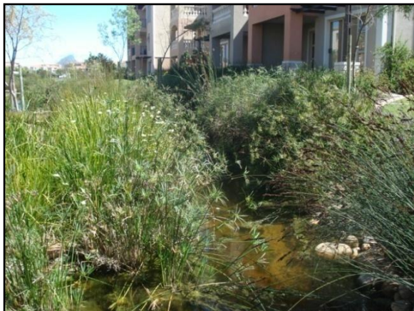
Figure 4.7: Pocket wetland at the low point of a residential complex
