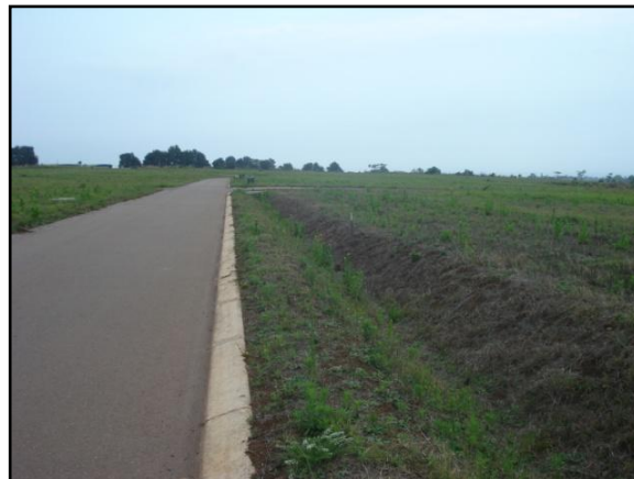
Figure 2.11: Enhanced dry swale, Cotswold Downs Golf Estate, eThekweni
