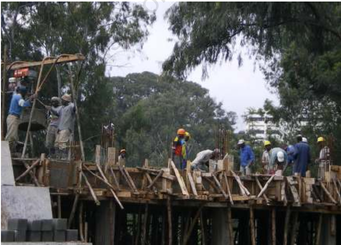
Plate 6: Concreting involves many craftsmen and trainees
