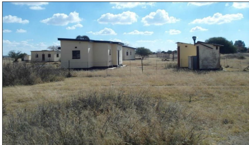
Optic formant 1.22. Pre-independence self-built housing units in Borolong. Source: Nkooe.
