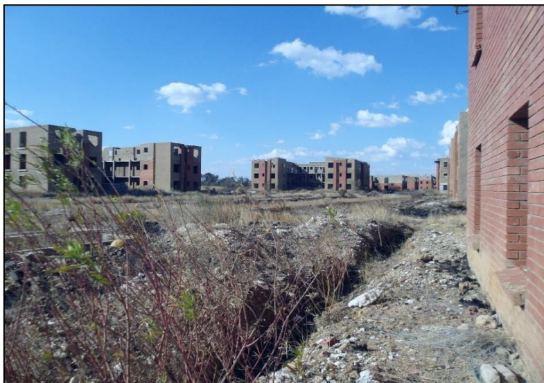
Optic formant 1.9. Incomplete low-cost housing construction in Mmabatho. Source: Nkooe.
