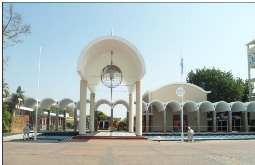
Optic formant 1.8. Parliament Precinct of the Republic of Botswana in Gaborone. Source: Nkooe.
