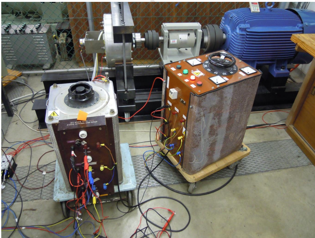
Figure 98: Dip Simulation Variable Transformers in Laboratory Setup
