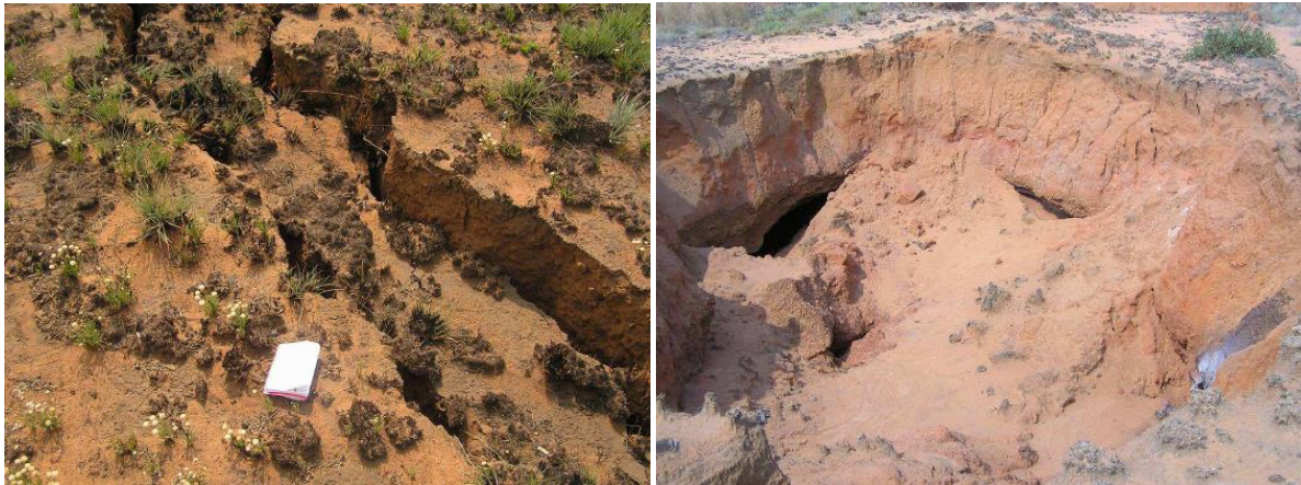
Figure 2-3: Tension cracks representing the primary impact of surface subsidence and a sinkhole also showing openings into underground workings (Heath and Engelbrecht, 2011)
