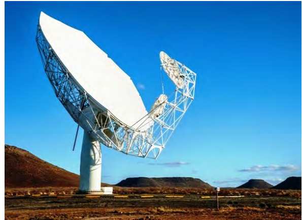
Figure 2.9: The first of 64 13.5 meter diameter dishes of the MeerKAT SKA precursor radio interferometer, completed in early 2014 [12]
