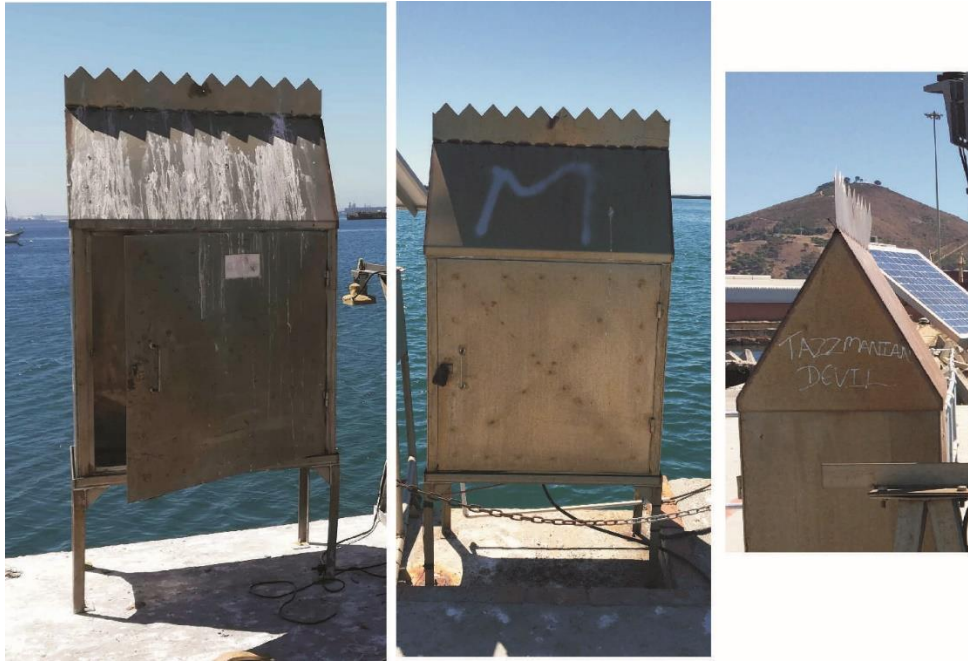
Figure 21 is the “bird proofing” on top of the tide gauge cabinets (2018).
