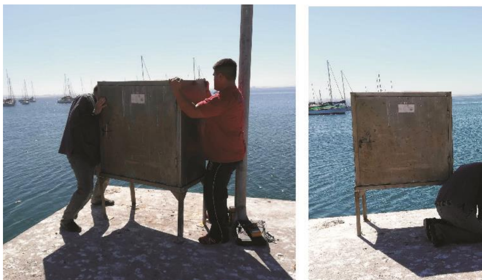
Figure 20 is a tide gauge electronics cabinet being reinstalled in Saldanha (2018).
