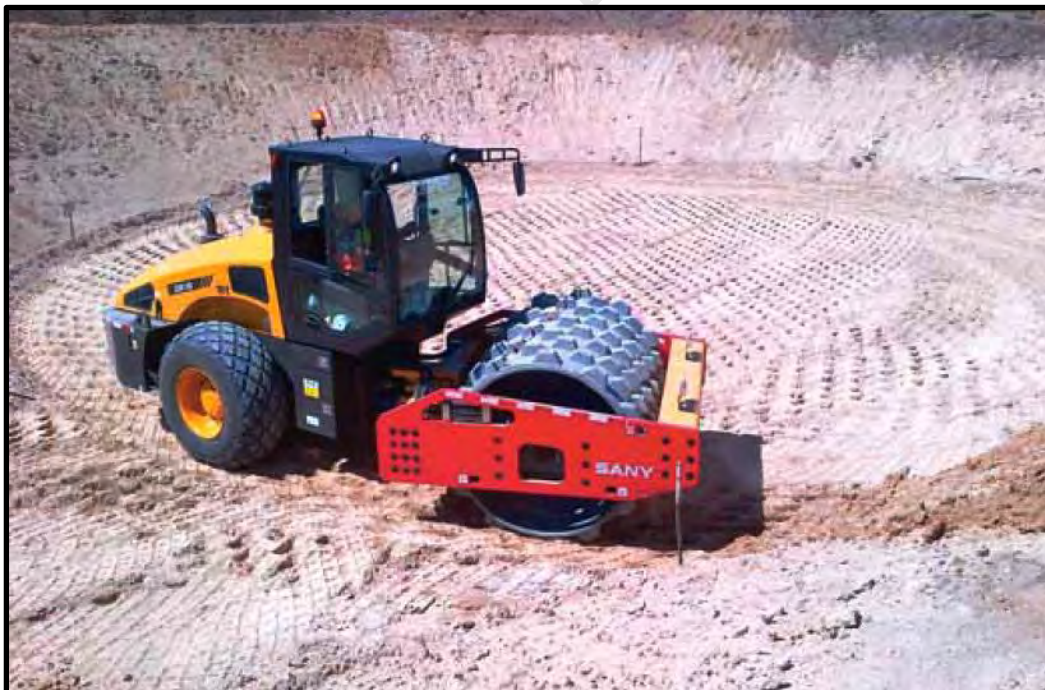
Figure 5.14 Vibratory roller compacting the surface of a wind turbine footprint (Parrock, 2013)
