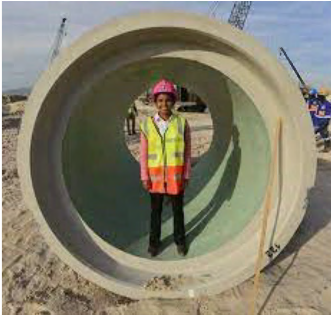
Image 3.5: Xanthea Limberg, Mayoral Committee Member for Water and Waste, at the Zandvliet Wastewater Treatment Works upgrade. (Source: https://www.bizcommunity.com/Article/196/604/192917.html )
