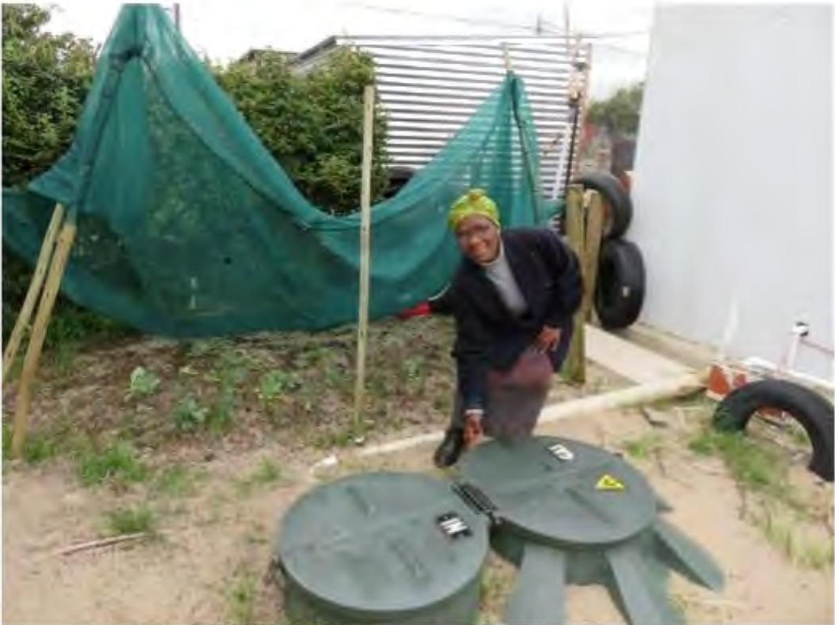
Image 6.1: Mam Wana at one of the community gardens at an Early Development Centre (EDC), where organic waste (including cow dung) is placed into a biodigester (pointed at by Mam Wana). The gas it produces is used for cooking and heating in the EDC. Decomposed material that settles at the bottom of the biodigesters is used as fertiliser. (Source: Author)
