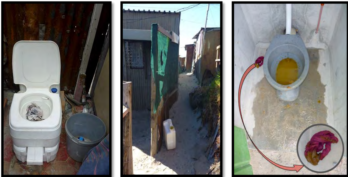
Figure 4: An un-sewered toilet in an informal settlement (left). The household unit is situated in an open space between two dwellings. The bottom tank is collected (centre), emptied and disinfected at a treatment works thrice weekly by a municipal service provider. Highlighted in the bottom-right inset is a rag that was used as an anal cleanser and discarded next to a blocked flush toilet (Taing, 30 January; 5 & 14 February 2013).
