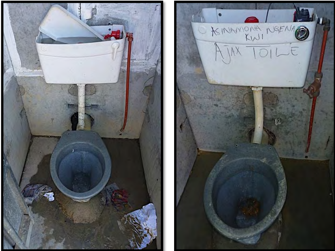
Figure 34: A toilet in ‘good’ (left) and ‘bad working condition’ (right) (Taing, 11 June 2013). While neither has seats or functional flush levers, my research assistant said the former is considered ‘good’ because it discharges waste as designed.
