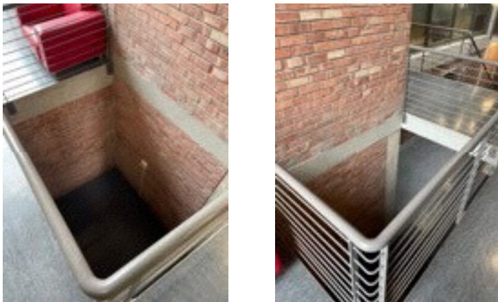
Figure 6. The elevator shaft in the New Building.
